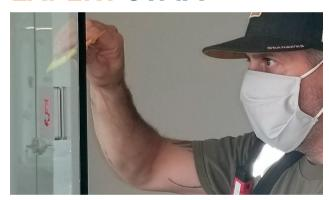
Expert installers placed all the signs with precision and attention to detail, including installing white vinyl on the inside of the glass to hide the mounting adhesive.
